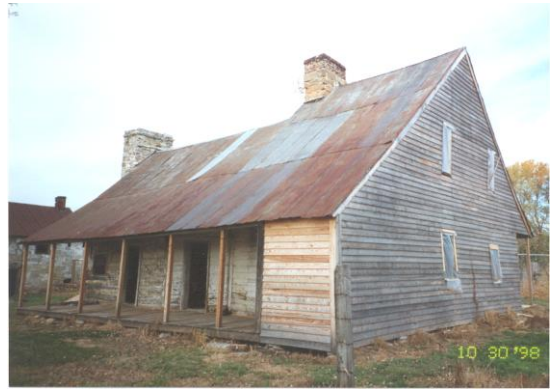
East Wall, Four Windows
