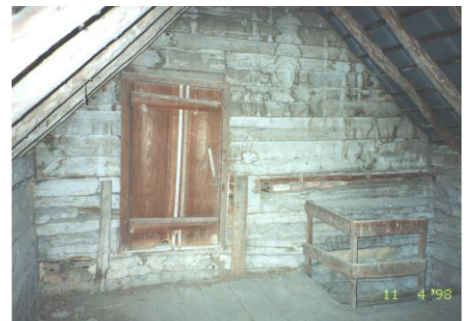
Loft, R205, east wall, D204, stair well.
