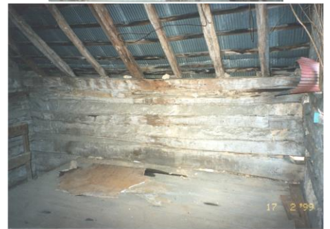
Loft, R205, south wall.
