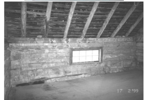
Loft, R205, north wall, W202.
