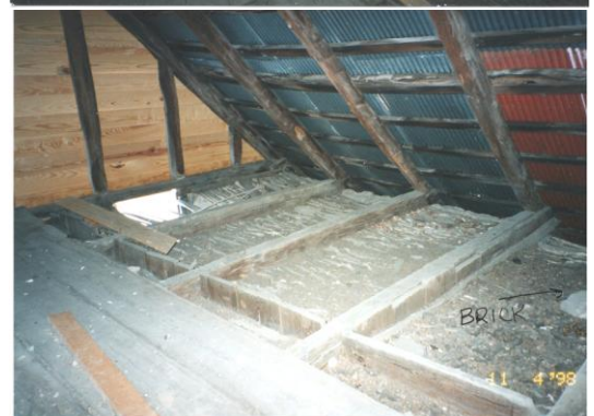
Attic over ca. 1751 Section, East and South
