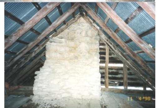
Attic over ca. 1751 Section, West Wall, Chimney Mass
